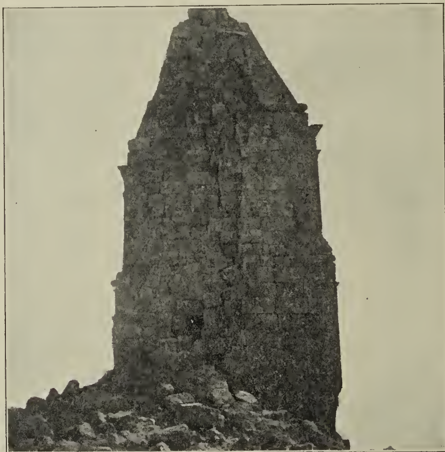
SOUTHWESTERN CORNER OF KAMU'AT HIRMIL, DESTROYED BY TREASURE SEEKERS
